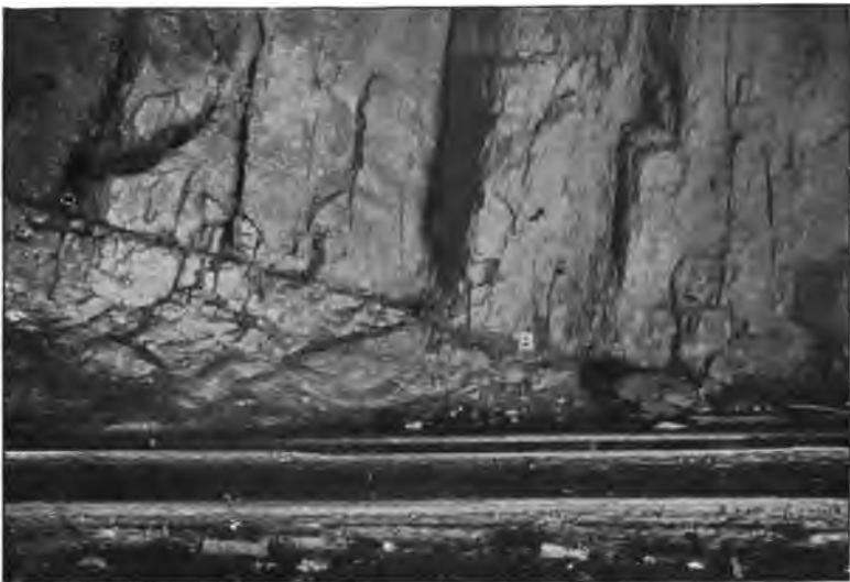
Fig. 2. Lower contact of Palisade diabase on sandstone (arkose), Pa. R. R. tunnels, Weehawken, 50 feet below mean high tide. The diabase exhibits the typical rectangular jointing. (Reproduced by courtesy of Chas. M. Jacobs, Chief Engineer.)
